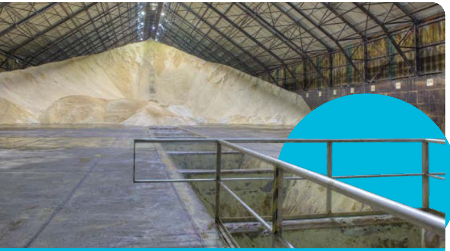
Bulk storage of sugar at STL's Mourilyan terminal.
